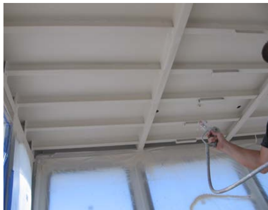
Figure 6 Commercial Application of Silent Running and TEMP-COAT to aluminum super-structure to reduce structure borne noise and control thermal loads. Photo Courtesy of TEMP-COAT Brand Products
