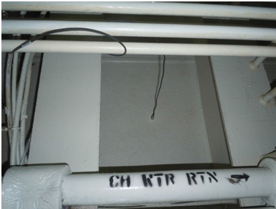
Figure 7. Accelerometer installation on structural bulkhead
