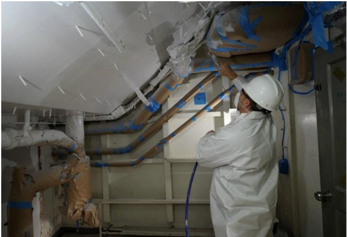
Figure 15. Damping installation on catapault trough
