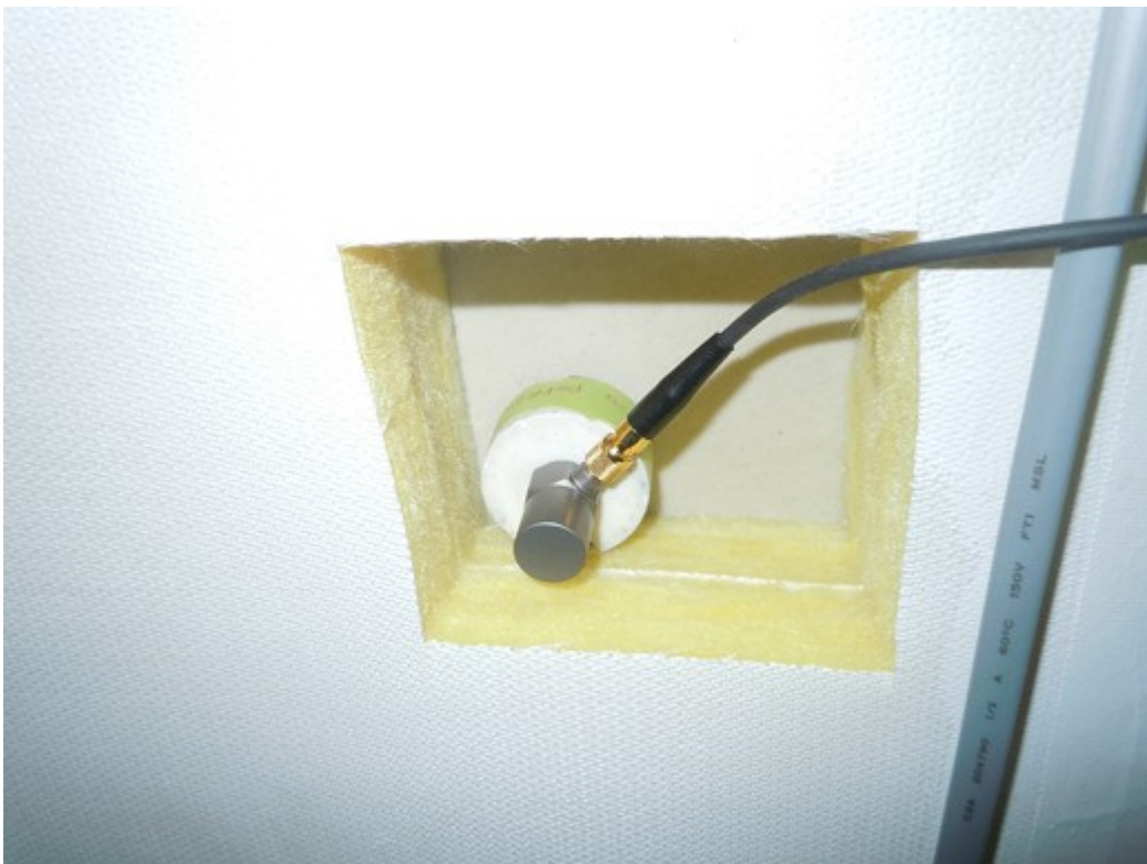
Figure 9. Accelerometer installation on catapult trough
