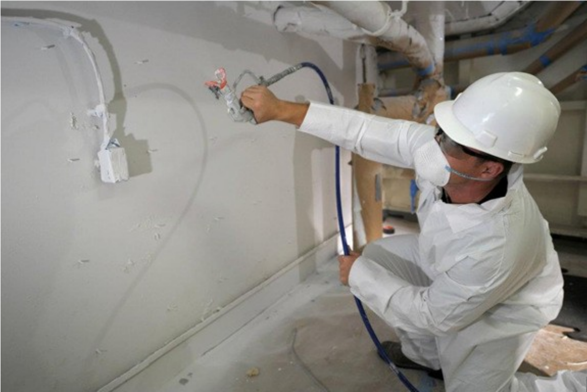
Figure 14. Damping installation on structural bulkhead.
